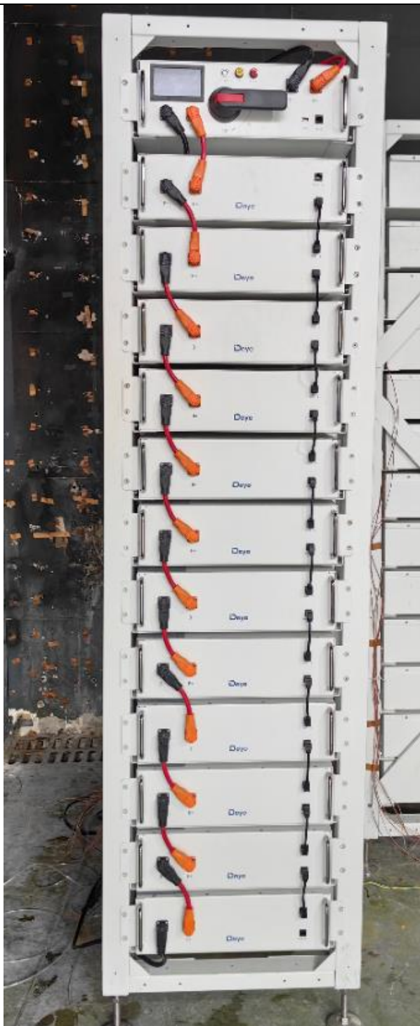
Figure 3a. External view 01 of battery system
