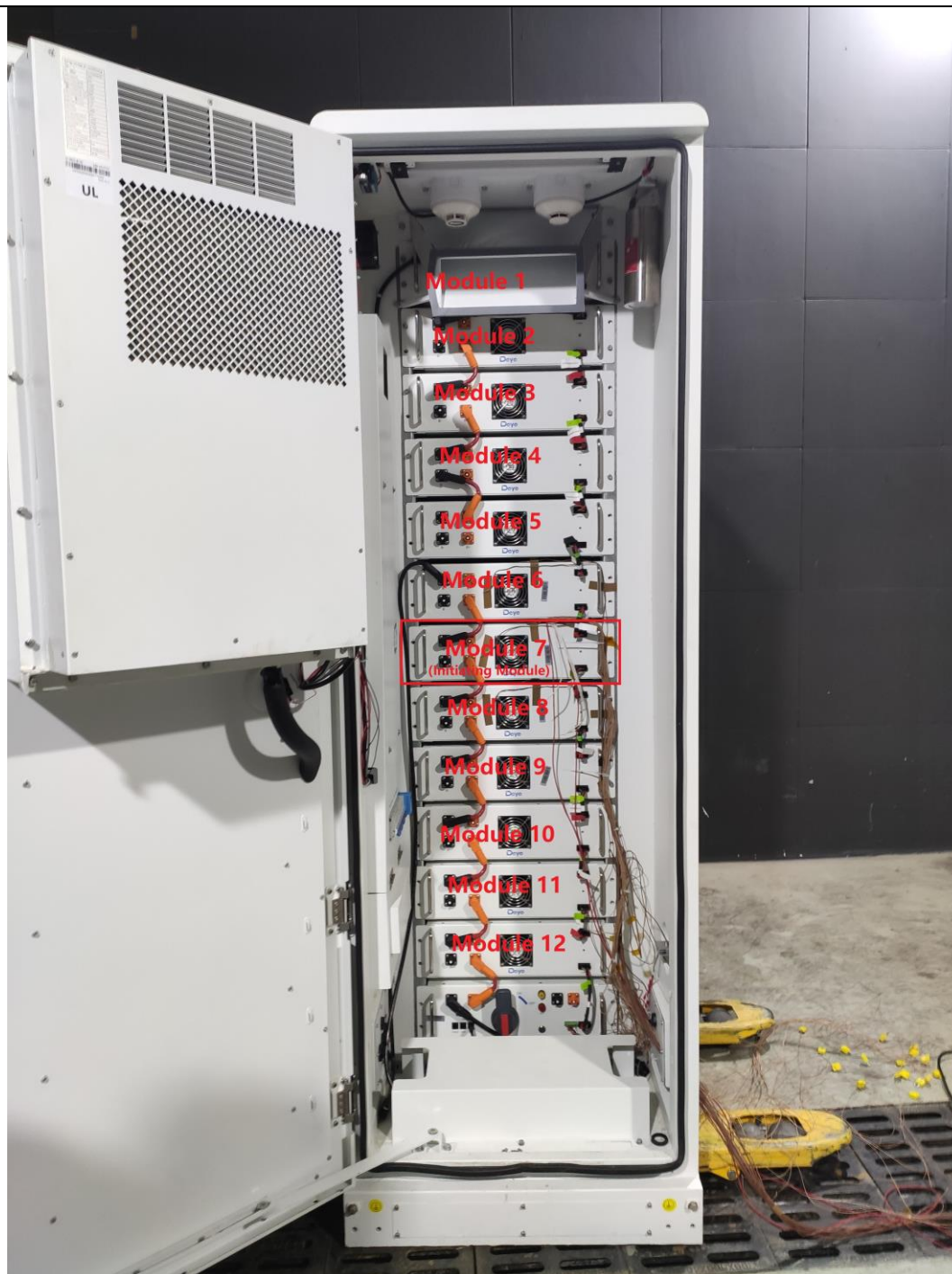
Figure 10c. View of initiating module in initiating BESS unit
