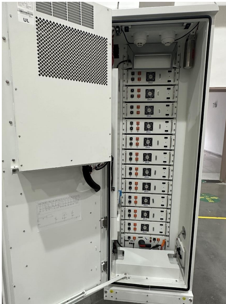
Figure 5. Internal view of battery unit (GE-FH60)
